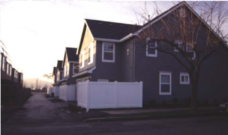
Buckman Heights Townhomes, Northeast Portland
