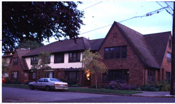
Rowhouses, Southeast Portland
