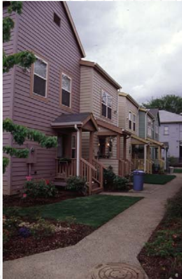
North William Townhomes, Northwest Portland
