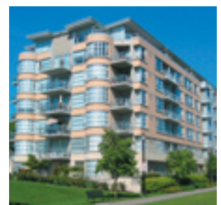
6 Story Multi-Family Residential in Vancouver
