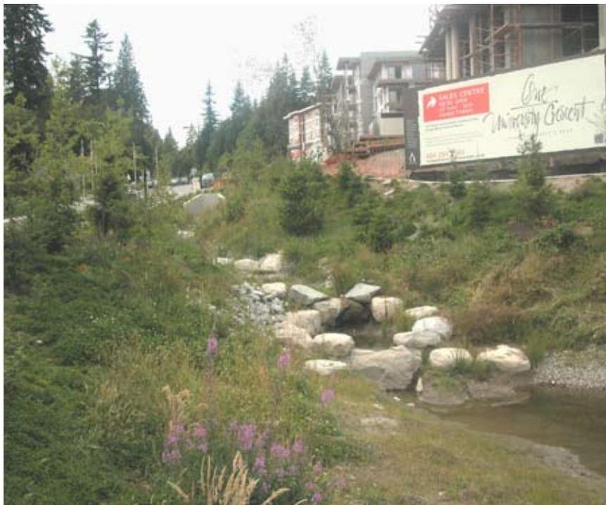
*Natural drainage systems in which stormwater is held on the surface and allowed to seep naturally into the ground protects against downstream degradation such as streambank erosion and increased water temperature, which is a byproduct of conventional stormwater management systems. Using natural systems to collect and filter stormwater reduces infrastructure costs. This neighbourhood protects all streams and uses natural systems for stormwater management.*
